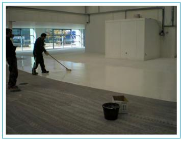
Epoxy undercoat and vinyl flakes are applied to the Stonclad 4mm mortar to enhance aesthetics, protection and slip resistance.
