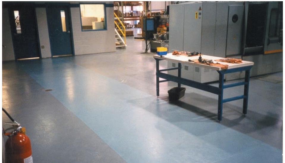
Stonhard's Stonclad PT sealed with Stonkote GS4 offers the chemical and abrasion resistance necessary in the harsh production area at Milan Screw Products.
