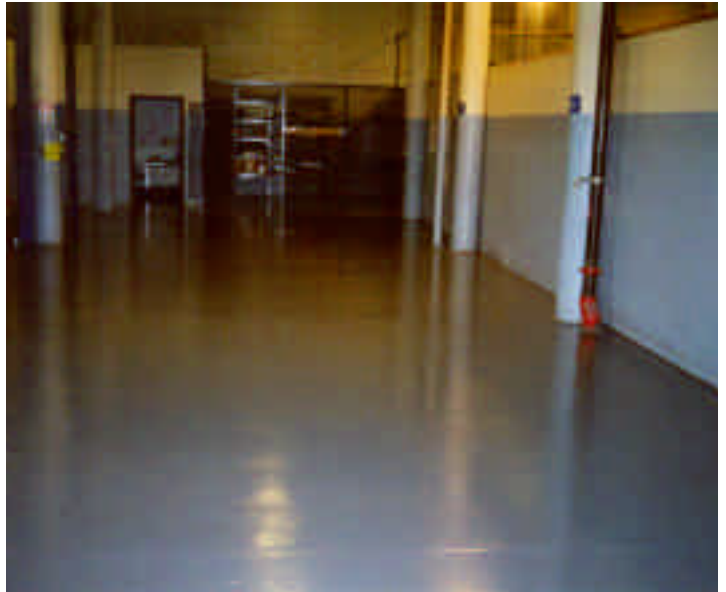
Stonhard's seamless system dramatically reduced on-going maintenance costs.
