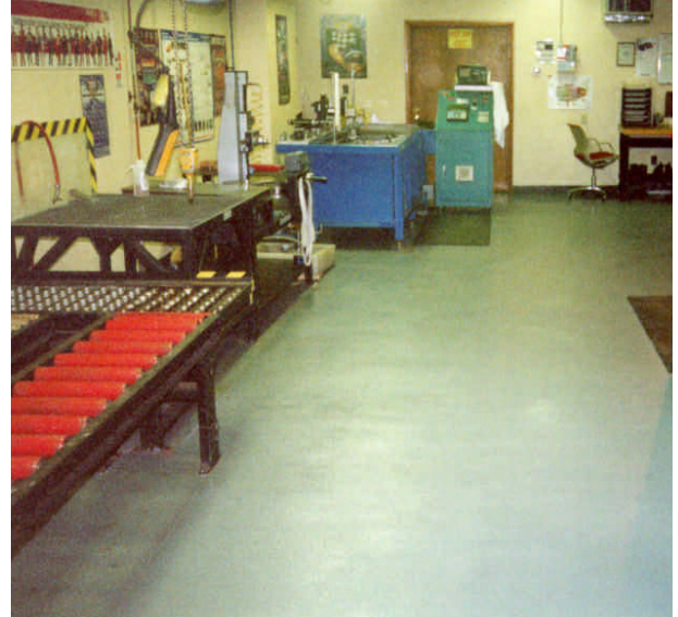
Failing concrete was repaired and coated with a durable, chemically resistant epoxy system. The facility is now a safe and attractive working environment.
